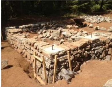
Fig. 1: Implementation of stone foundation
